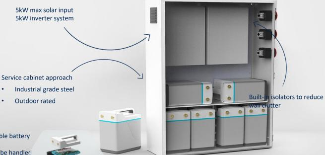
5-11kWh of removable battery modules (module weight can be handled by 1 technician)
