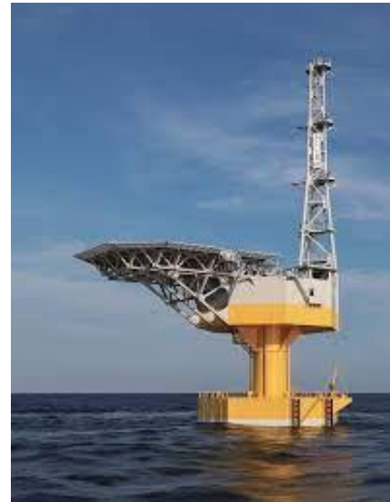
Figure 14. 66kV substation "Fukushima Kizuna", Courtesy of Fukushima Offshore Wind Consortium. 3
