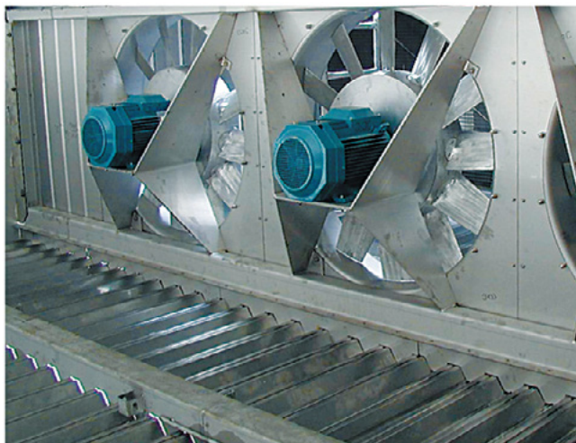
"Motors with axial fans in ventilation system" Supplied courtesy of Siemens
