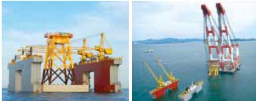
Figure 72. Installation of hybrid gravity/jacket structure in Kitakyushu (NEDO, 2013)
