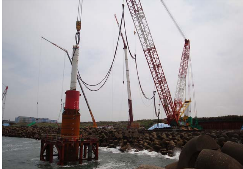
Figure 77. Installation of monopile using onshore crane at Kamisu nearshore wind farm (Moricho, 2010)
