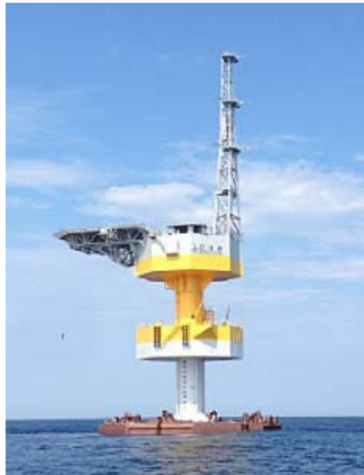
Figure 26. Fukushima “Kizuna” 66kV floating sub-station (Shimizu Corporation, 2013).
