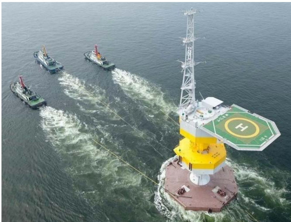
Figure 78. Floating substation for Fukushima demonstration project being towed out to site using simple tug boats (Renewables International, 2013)
