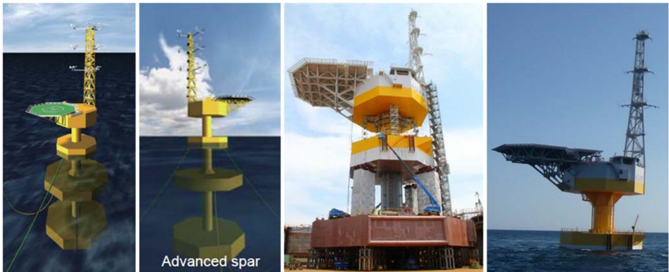
Figure 62. Japan Marine United's Advanced Spar with substation at Fukushima (Fukushima FORWARD, 2013)
