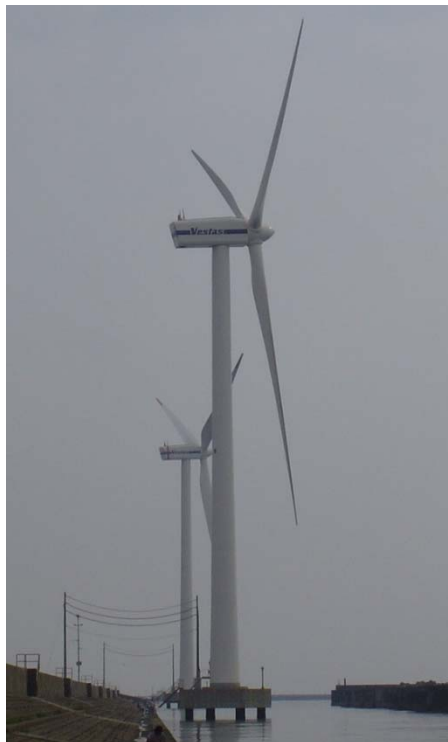
Figure 52. High-rise pile cap foundation supporting 2 MW turbine at Sataka nearshore wind farm (Wikimedia, 2005)
