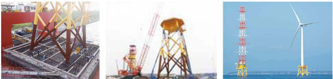
Figure 55. Hybrid gravity/jacket foundation installed at Kitakyushu demonstration project (NEDO, 2013)
