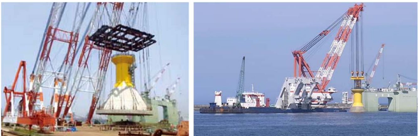
Figure 71. Installation of gravity-base foundation at Choshi (TEPCO, 2014)
