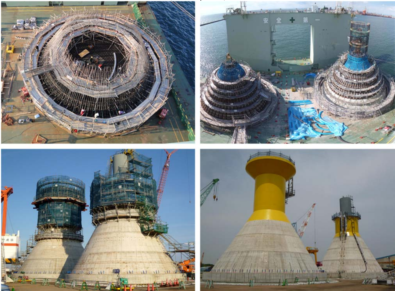
Figure 54. Fabrication of the gravity base foundation installed at Choshi demonstration project (TEPCO, 2014)
