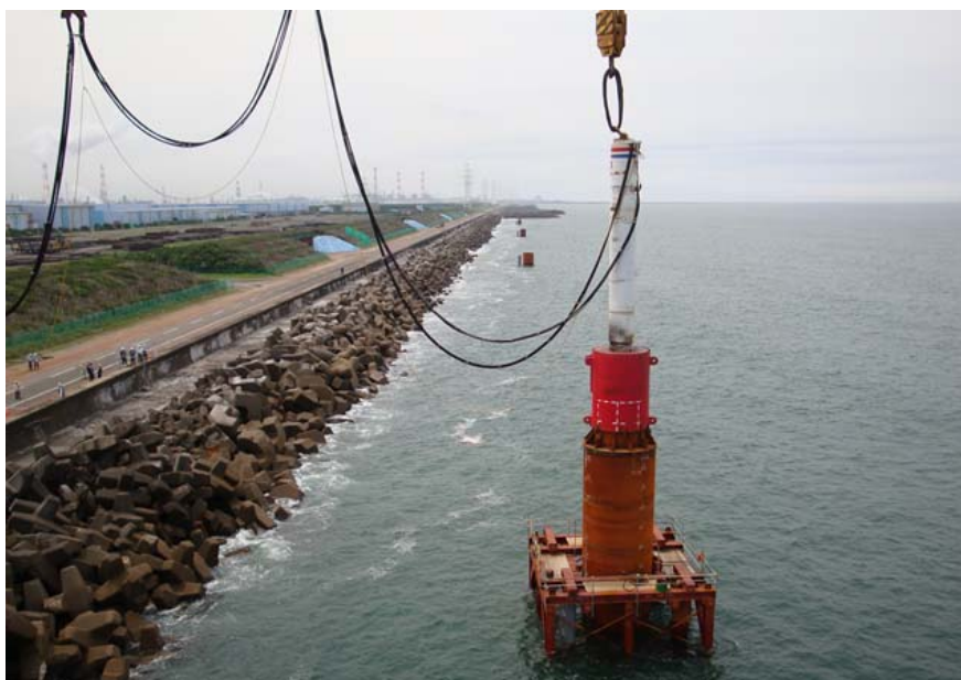
Figure 69. Piling hammer installing a monopile foundation at Kamisu nearshore wind farm (Moricho, 2010).
