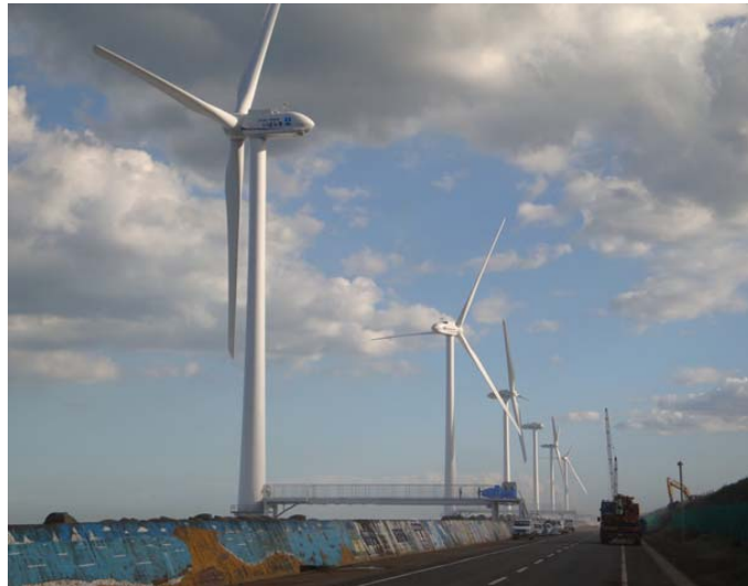
Figure 80. Gangway access from land to nearshore turbine at Kamisu nearshore wind farm (Moricho, 2010)
