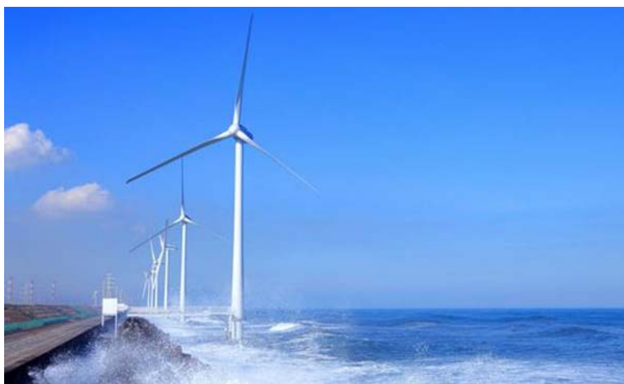
Figure 53. Fuji 2 MW turbines installed on monopiles at Kamisu nearshore wind farm (New Energy News, 2011)
